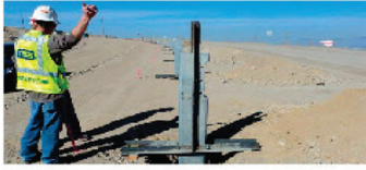
Utah Data Center, Texas
