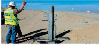
Utah Data Center, Texas
