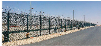
New Sudair 380kv substation, KSA
