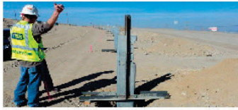
Utah Data Center, Texas
