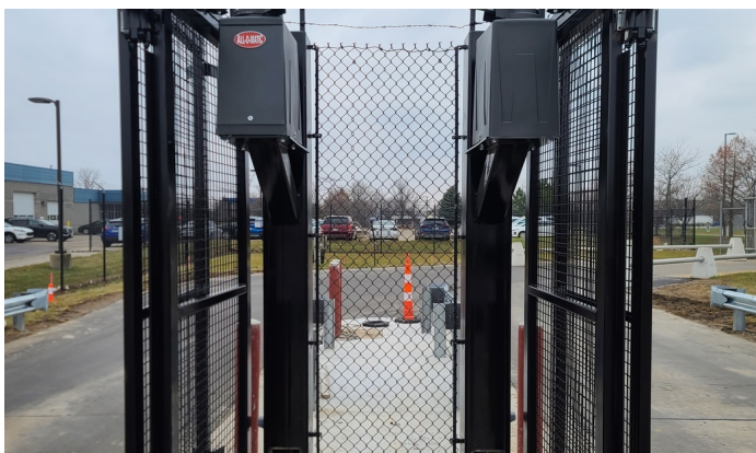
Post-mounted drive and hinge assembly.
