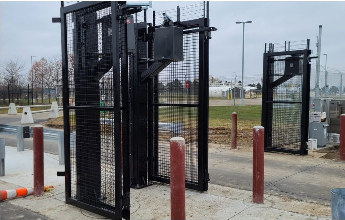
Mesh infill on a cantilever system, gate open.
