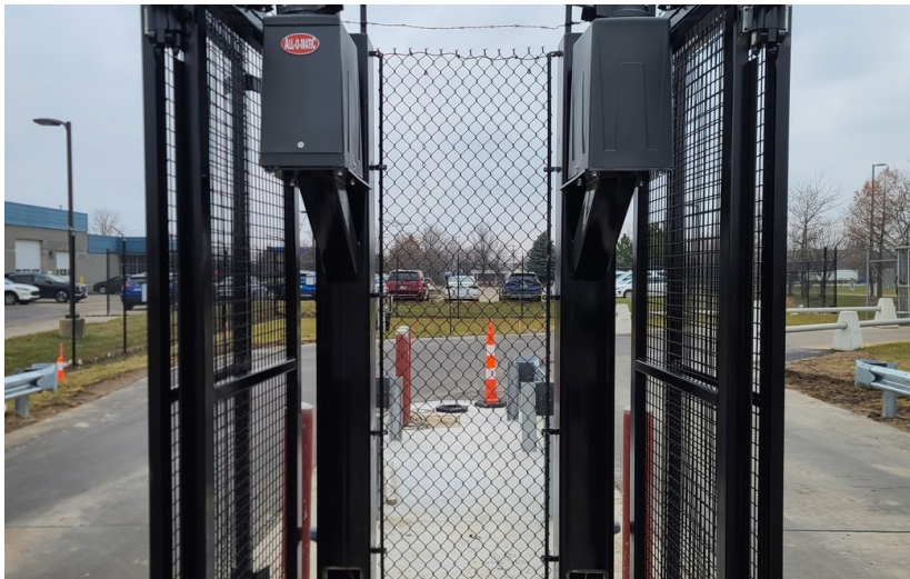
Post assembly and drive, set on its pier at the edge of the lane.
