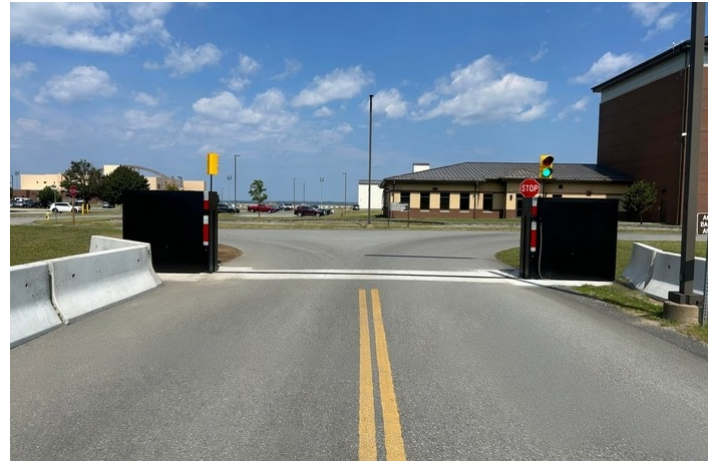
Retracted — the same entry point, net down in the pan and flush with the surface. Traffic crosses it without slowing.
