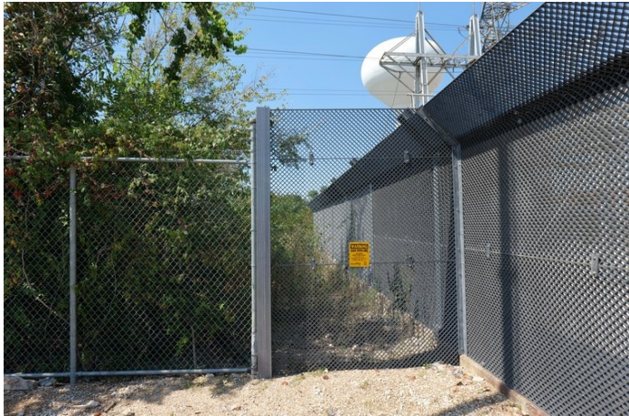
ENC fence running to a chain-link tie-in — the two systems can share a line.
