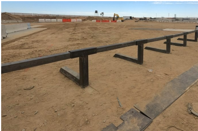
A finished run at the crash-test facility — three 42-foot spans joined end to end through the ballast.
