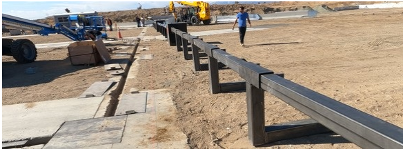
Spans running end to end — the same parts repeated to whatever length the opening needs.
