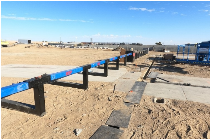
A run set straight onto a graded surface — no anchors, no core holes, nothing below grade.
