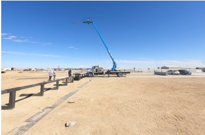
A completed run alongside the plant that set it — a forklift or a boom truck is the whole equipment list.
