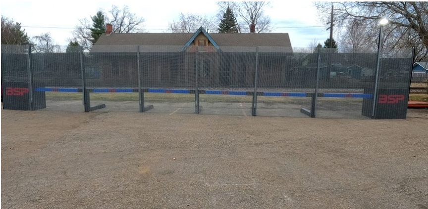
Vehicle barrier and anti-climb pedestrian barrier carried on one frame. The acrylic shield mounts to the same posts, on the protected side.
