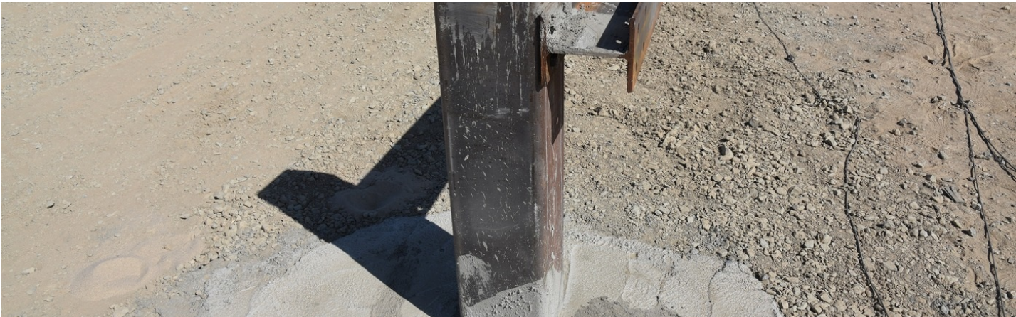
Post and beam under construction at the proving ground — beam seated on the crash post.
