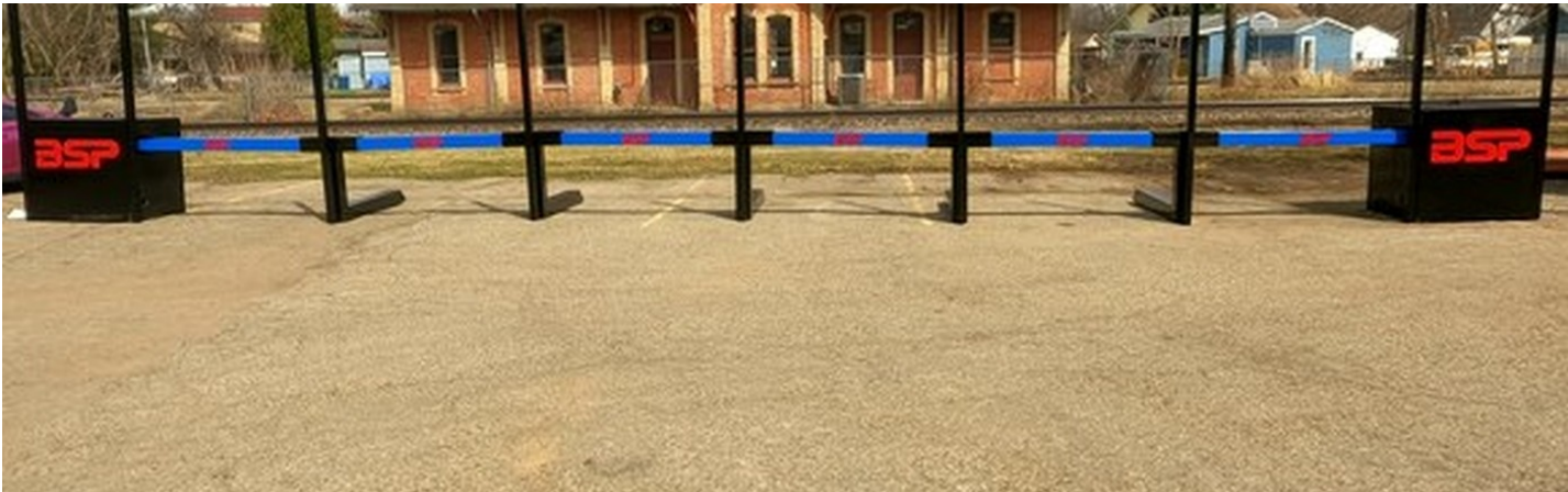
MPPD run deployed on grade. No foundation, no excavation, no permanent works.
