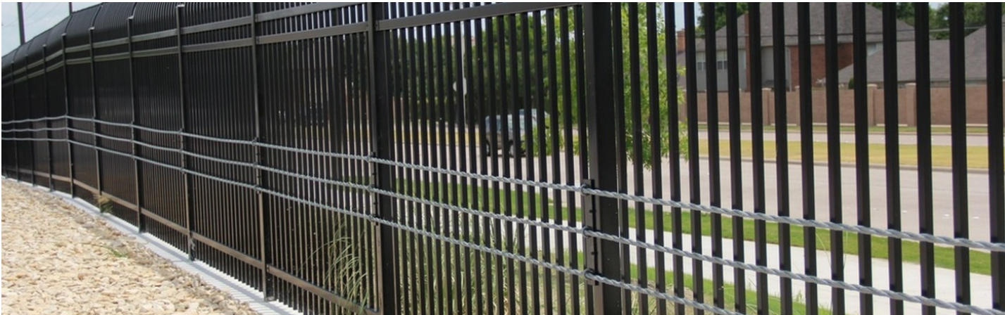
Passive cable line carried behind an ornamental fence — the barrier is invisible from the approach.
