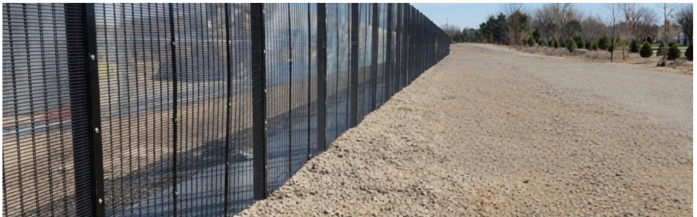
SecureMesh at a corporate perimeter — near-transparent for cameras, finger-proof to a climber.
